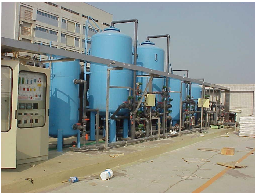
The full scale ion exchange system for copper removal. Capacity=30m 3 /Hr (WUS Printed Circuit, Taiwan)
